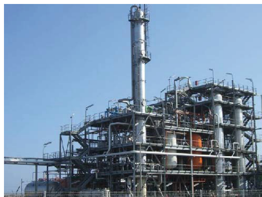
Fig. 3. Diester Industrie Esterfip-H biodiesel facility in Sète, France.
